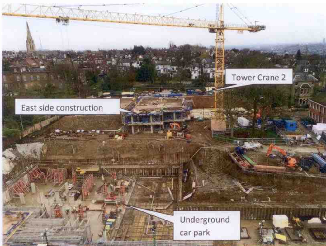
Current view from Tower Crane 1
